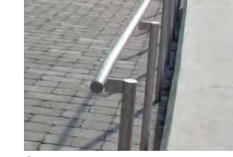
Stainless steel handrail
